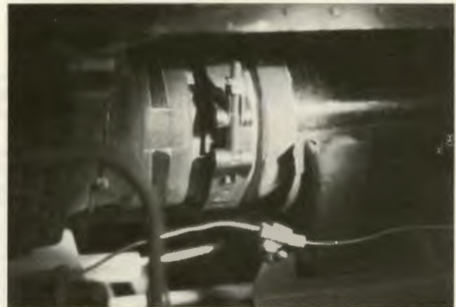
IMPROPERLY INSTALLED CLAMP
